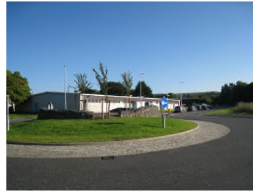
View towards Business Park from Railway Terminus
